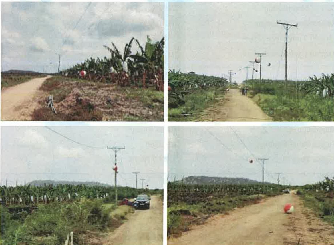
Figure 2: Damaged Power line
